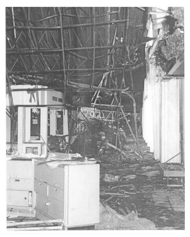
**Photograph** 6. Moving further east in the covered mall, the counters in the foreground are also in Photograph 3. This area is where the metal roof began a partial collapse. The goods in the kiosks were either stored before the fire or removed prior to the picture.
